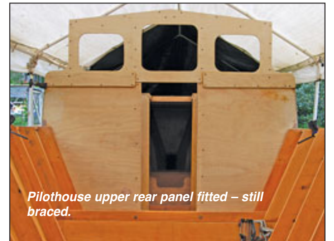
Upper aft panel for the pilothouse.
