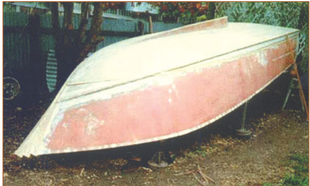
Above: The hull with the new ply and keel fitted and ready to be turned up the right way.
