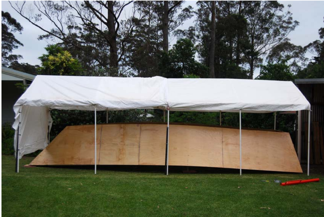
Temporary carport structures for site cover
