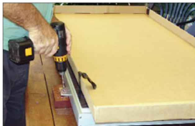
Installing the solar panels is relatively simple. The underside of the frame is pre-drilled, and because the maker's recommend that you don't install the panel (and its all-important electrical controls) hard onto the roof, we prefer to lift it up about 20-25mm so that it sits clear of the roof - and rain or hose water can then pass harmlessly underneath.
