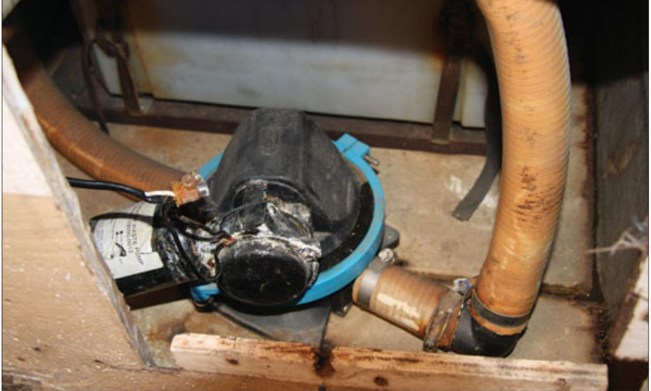
better appraisal of suitable cable size. Similarly considerations apply to the macerator (rated at 20 amps and stall current at 70). I determined (from tables) that the recommended size for the current and distance in this instance was 13 to 21mm sq. to limit volt drop to 3%, or 5 to 8mm sq. for a 10% drop! I would probably have used 6mm sq. or, more likely, found some 13 or 16mm sq. giving me something in between 3% and 10% - like I said, mostly common sense.
