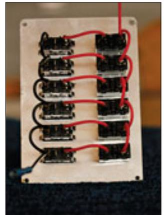
on simultaneously. In this instance there were 3 searchlights, a shower pump, bridge lights, deck lights and "Aux." Consider the positive "bus" on the back of this panel – looped in and out of each breaker, in what seems to be less than 1mm sq. wire!
