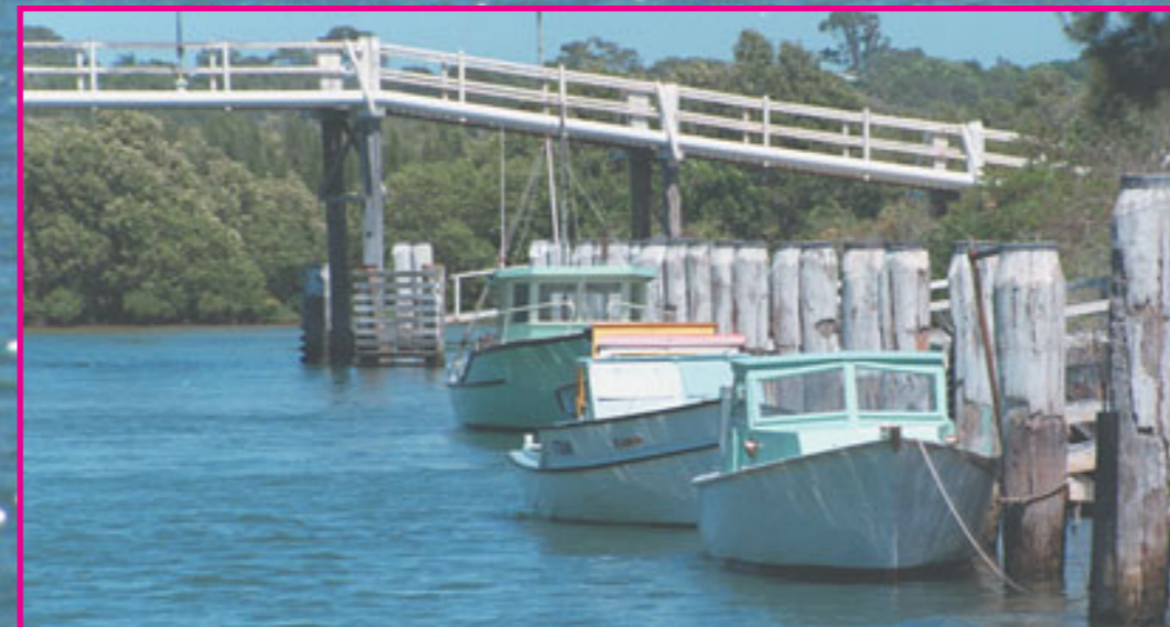
Back Creek moorings
