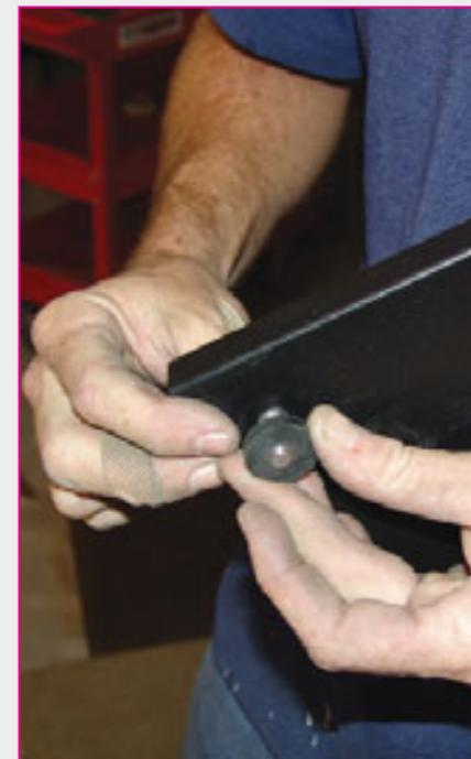
checking what you have planned. Note he has texta-marked the base plate's position first. Next, Mick pushes the base plate washers onto the screws, noting that these washers
